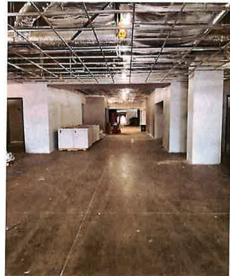
1 st Floor Ceiling Grid, Drywall, & Paint
